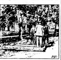
REGULATING THE DRAG BY STEPPING ON IT, CENTER OF THE ROAD. ONE TRIP WILL ANSWER, BUT ANOTHER ONE OR TWO WILL HASTEN MATTERS. AFTER THE NEXT TRIP DRAG IN THE SAME MANNER, AND FOLLOW UP THE THIRD, FOURTH AND FIFTH TRIPS, WHEN THE CENTER OF THAT PORTION OF THE ROADWAY YOU HAVE BEEN DRAGGING WILL BE THE HIGHEST. IT MAY BE EITHER NARROW, IF SO, PLANT ONE SHALLOW FURROW ON EACH SIDE OF THE DRAGGED PORTION, TURNING THE FURROW IN THE ROAD. SPREAD THIS LOOSE EARTH OVER THE ROAD WITH THE DRAG. THIS OPERATION THE ROAD HAS BEEN WIDENED ABOUT TWO FEET. FLOW NO MORE UNTIL AFTER ANOTHER RAIN. FLOW AFTER EACH RAIN UNTIL THE ROAD IS WIDE ENOUGH TO SUIT YOU. IF YOU FOLLOW THIS PLAN YOU WILL HAVE A GOOD SLOTTED ROAD FROM THE BEGINNING. THERE WILL BE A MINIMUM AMOUNT OF MUD AND DUST, THE CENTER OF THE ROAD WILL BE ALWAYS FIT FOR TRAVEL, AND YOU CAN BUILD THE GRADE AS HIGH AS YOU WISH. THE ROAD WILL BE VERY MUCH BETTER FROM THE BEGINNING, BUT IT WILL NOT REACH ITS HIGHEST STATE OF EFFICIENCY UNTIL IT HAS BEEN DRAGGED REGULARLY FOR FOUR OR FIVE YEARS.
