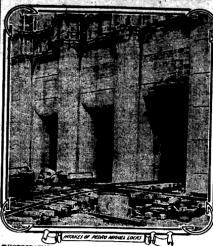
PHOTOGRAPHS just received from Panama show the progress that is being made on the great canal. The one here reproduced shows the intakes of the center wall, north end, of the Pedro Mixuel locks. These intakes are eight feet by its and admit water his the 1s-foot culteret in the center wall.
