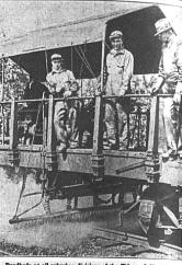
Roadbeds on all suburban divisions of the Chicago & North Railway and on the main lines between Chicago and St. Paulot lis and Chicago and Omasha are being oiled in a program started to give patrons dust-free travel on that line. The above picture side oiler in operation. The oil is heated and put conto the roadbed un
