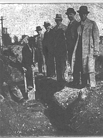
Village trustees inspect the fruition of several years' work in planning an adequate sewer system for Barrington. The group is shown above surveying work being done on East Hillside avenue. They are (reading left to right): Trustees Rudolph Kocher, John H. Blanke (resigned from board since photo was taken), John J. Carroll, H. D. A. Grebe, Village President Earl Hatje, Newton O. Plazge, and John F. Dueschler.
