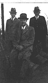
(Left to right)—Village President Earl Hatje and Village Trustees John F. Dueschler and H. D. A. Grebe pause for a moment on their inspection tour of the sewer system to have their picture taken and enjoy a short rest from pressing village affairs.
