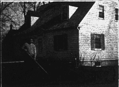
E. M. Schwemm has been one of the most active residents in the village undertaking construction work. Last year, two homes were completed for him and he is remodeling a third place on Summit street at present. He is shown above at the residence erected on Liberty street.
