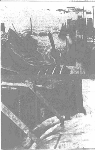
Above are two pictures showing the water rushing through the gap in the dam at Caesar Lake Sunday. The pictures were taken a few hours before the flood reached its peak, and show part of the spillway and timbers used in attempting to halt the flow.
